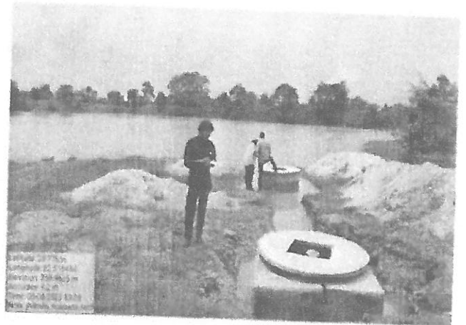
Percolation Ponds with Recharge Wells
