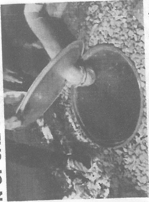
09) Fixing with Jali at top to avoid penetration of dust particles in side from top covering
